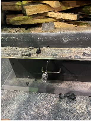
Air inlet mid-point setting for medium burn rate
