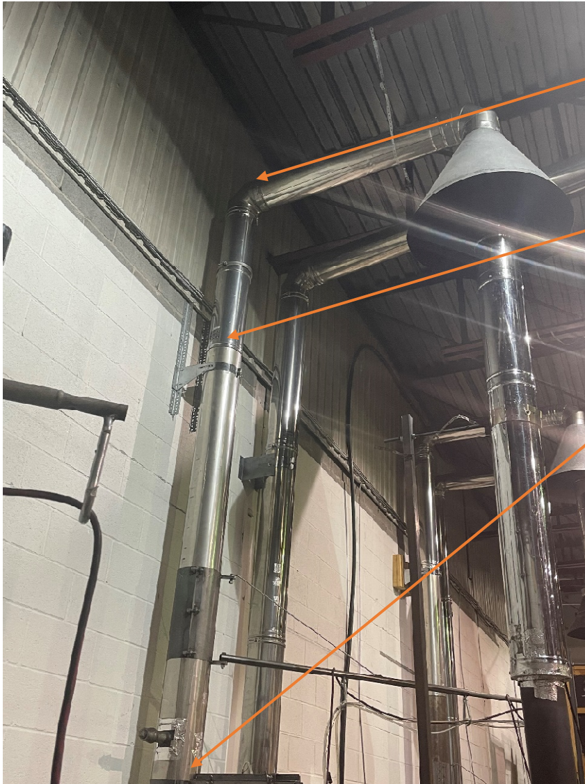
Total length between hood and sampling port: 29 feet.
