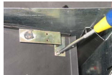
Figure 9 Fix temperature sensor bracket with two screws.
