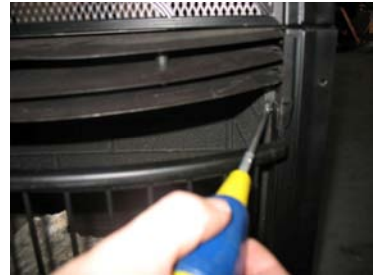
Figure 12 Unscrew two screws on the grill, remove the grill and logs.
