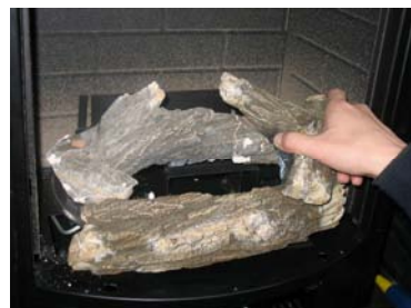
Figure 18 Lay back the logs according to the original layout.
