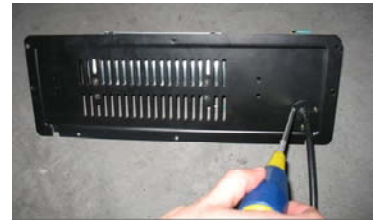
Figure 3 Fix and lay out the wires onto Blower Access Panel.
