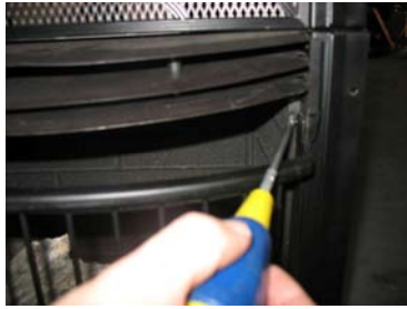
Figure 19 Re-fix the grill with two screws.
