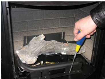
Figure 13 Unscrew the control panel (two screws) and pull it out a little bit. Notice: Pay attention not to loosen the igniting wire.
